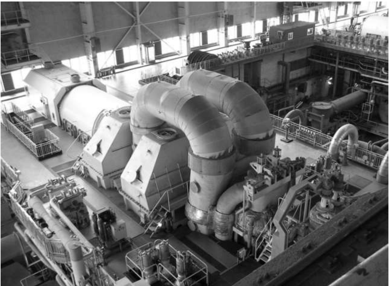
Figure 5. The object of study – a turbogenerator (turbogenerator with the capacity of 500 MW) responsible for producing electrical energy 4 (source: photo by Elektrownia „KOZIENICE” S.A. )
